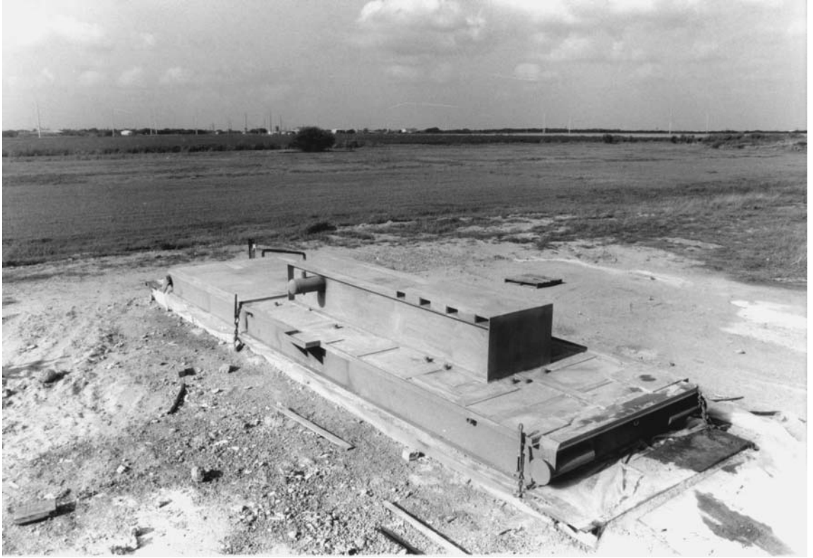
FIGURE 23.2 Typical skid design with concrete fill.
